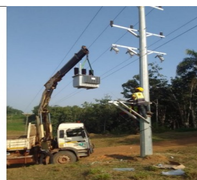
Transformer Installation Ongoing
